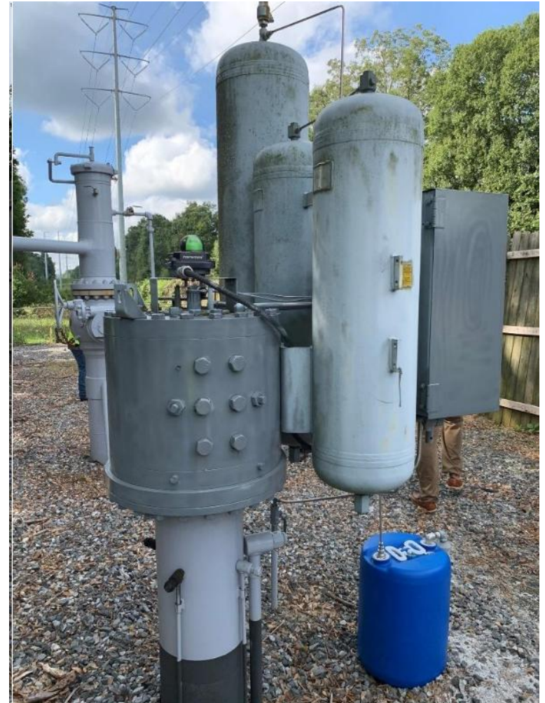
Gas over Oil Actuator
