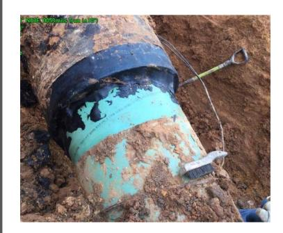
Filled Casing with Hot-Applied Fill-Coat #1Casing Filler
