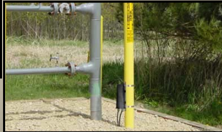
SSD – Solid State Decoupler
